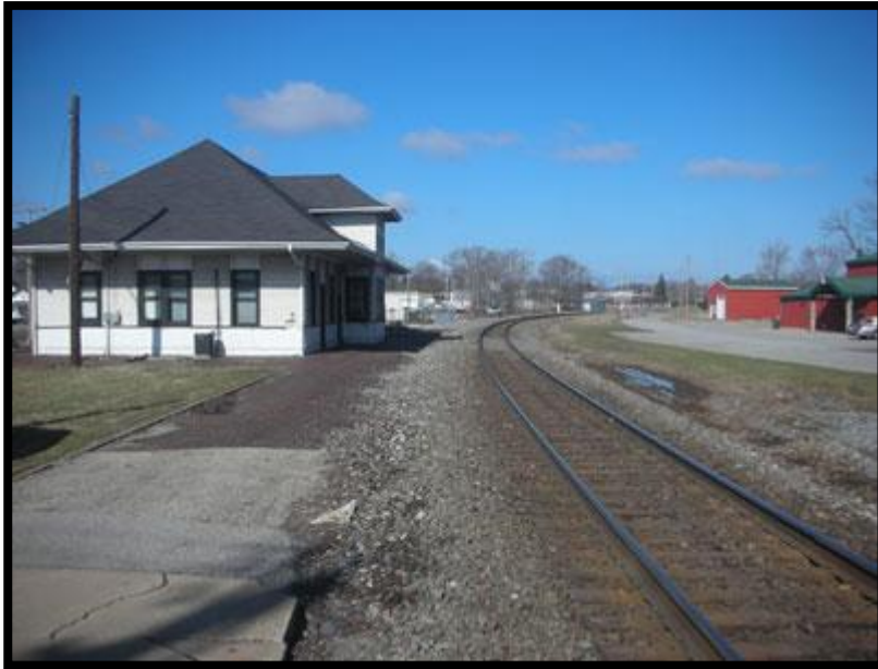
Former Location of the 1912 Grand Trunk Passenger Terminal
