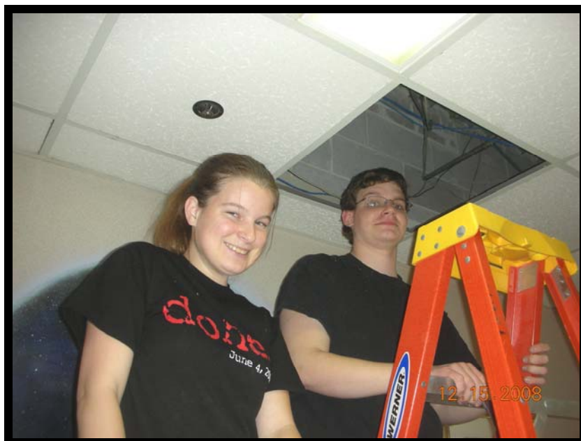
Electronic students spend some time learning about wiring internet, telephone, and television connections at the Career and Tech Center. Second year students (above), Stephanie Pucka (Hebron) and Matt Barney (WTHS) are seen above pulling wires for a new video line between our television studio and the televisions in the Commons.
